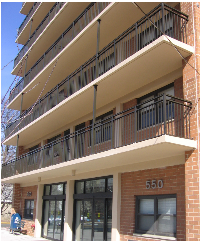
Overall view of the new railings.
