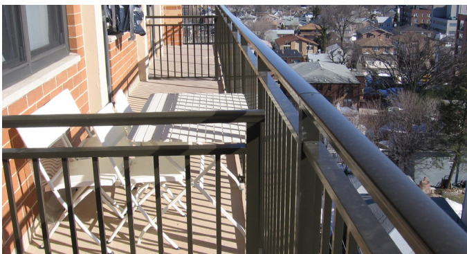
A view of the renovated balcony deck.
