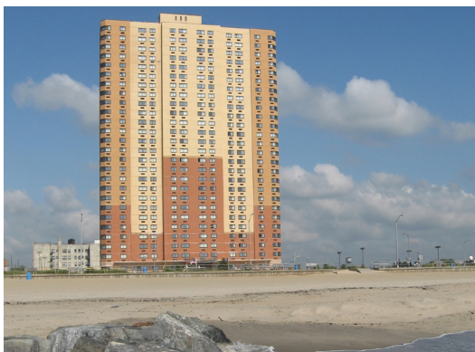
A view of the completed facade restoration.
