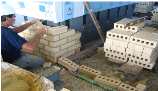
A photo showing the masonry being installed.
