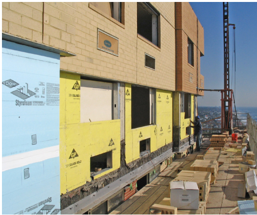
A photo showing the wall panel installation.
