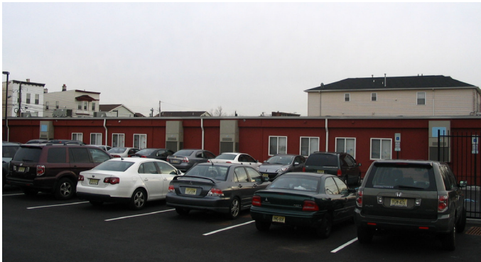
New parking lot at side of Classroom Building.
