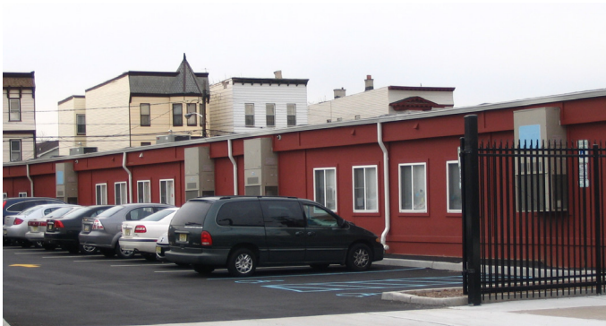
Gated front entrance to on site parking.
