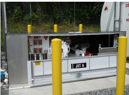
A view of the jet fuel pump and filtration system at Aeroflex Airport in Andover, New Jersey.
