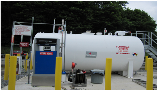
A view of the aviation gas tank and dispenser at Aeroflex Airport in Andover, New Jersey.
